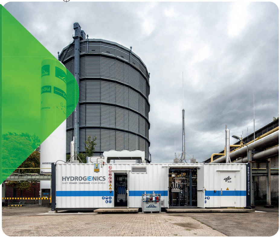
Container-integrated PEM electrolyzer linked to a H 2 refuelling station used at DLR for grid service testing
